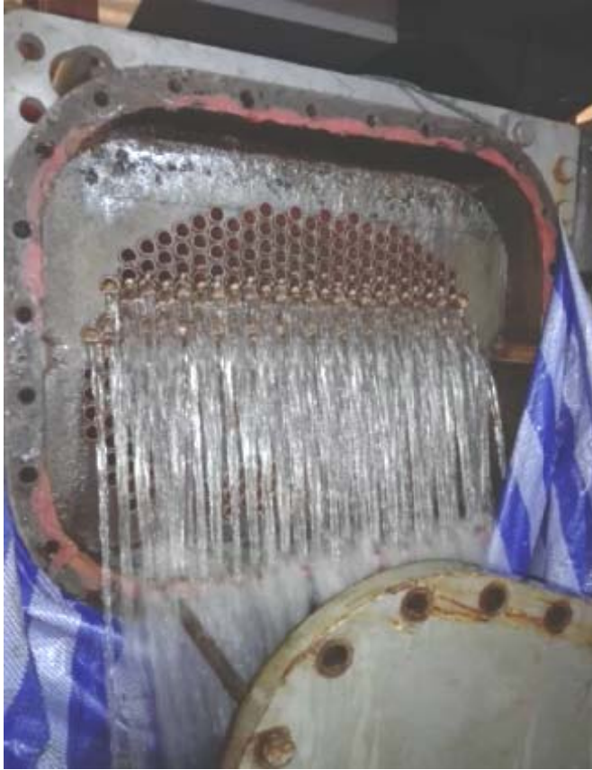
FLUSHING CONDENSER TUBE AFTER CLEAN SUCESSFULLY
