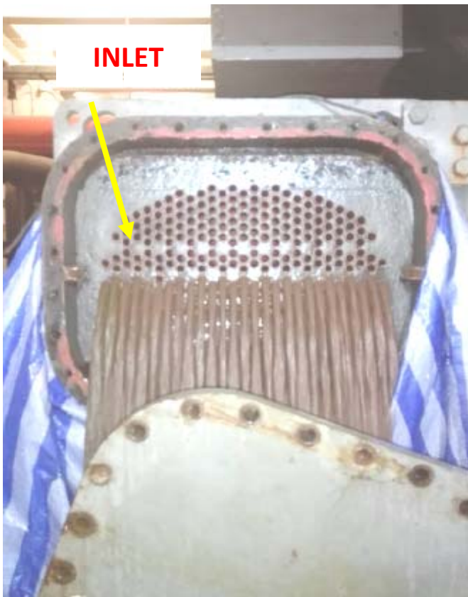
FLUSHING CONDENSER TUBE AFTER CLEAN SUCESSFULLY
