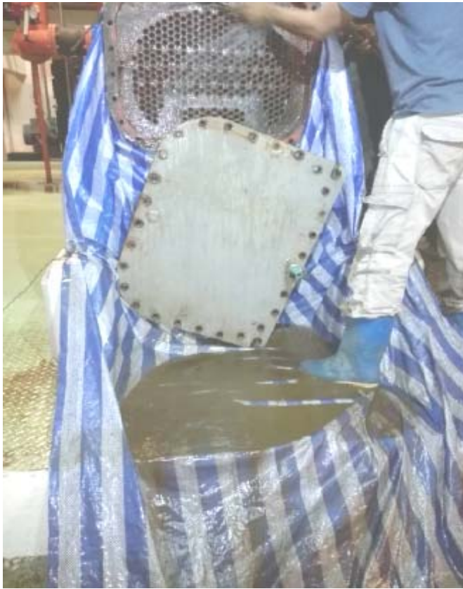
CLEANING SURFACE CONDENSER TUBE WITHIN CONDENSER LID
